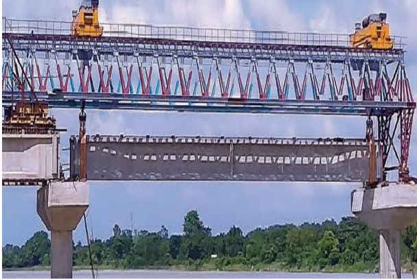
Steel Girder Bridges
