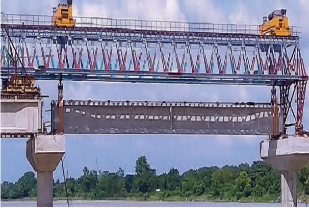
Steel Girder Bridges
