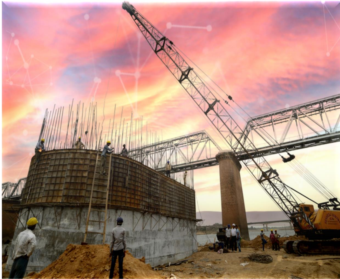
Kalpi Project Constructing railway bridge
