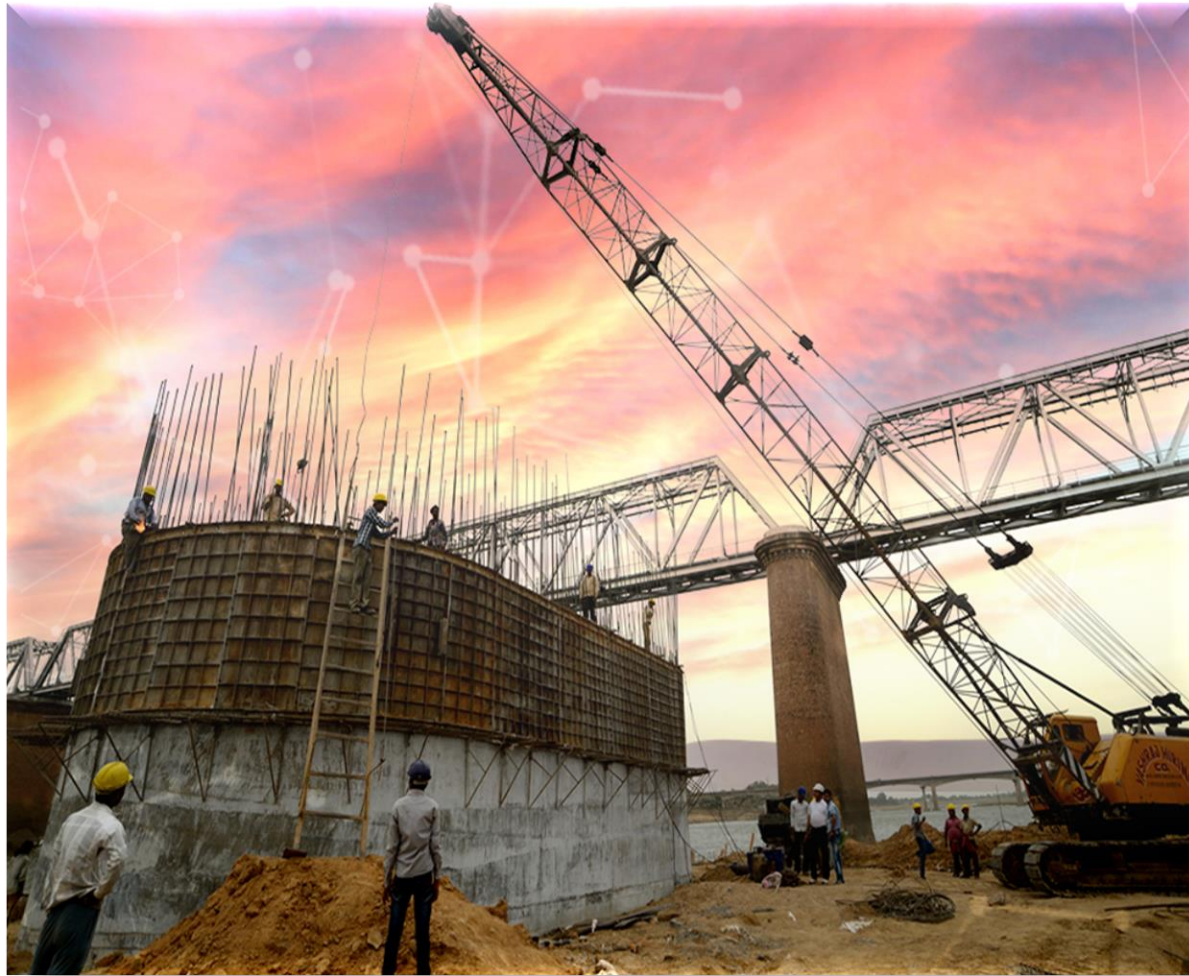
Kalpi Project Constructing railway bridge
