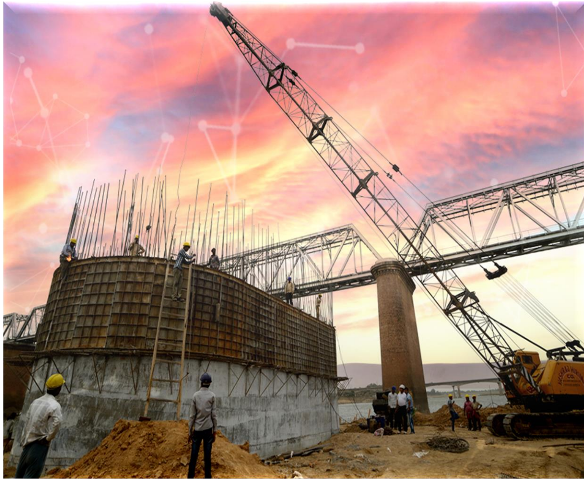
Kalpi Project Constructing railway bridge
