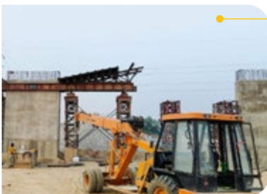
Constructing a bridge over Sangam in Allahabad
